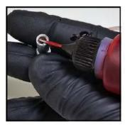
**31**Place a drop of red loctite (262) into anchor bolt
